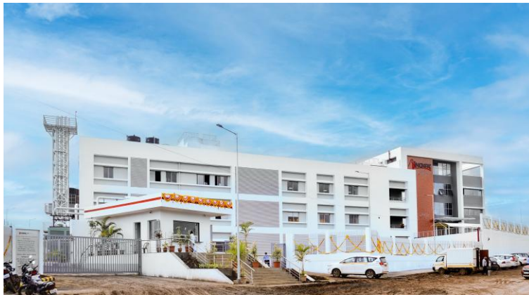
Inoxpa - New headquarter in Pune (India)
