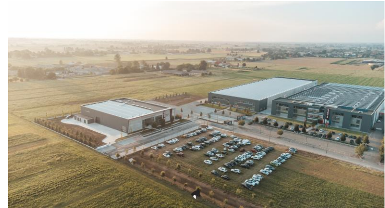
Walvoil – Factory extension in Cavriago (Italy)
